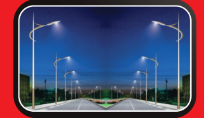
Underground Electric Connection
