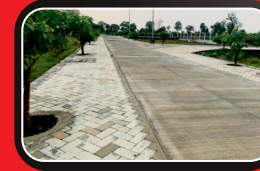
Internal Concrete Road
